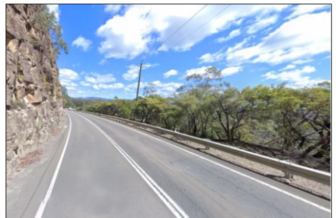
17. The drop associated with the Kurrajong Fault on the Bells Line of Road, Kurrajong Heights. (Source: R Miller modified from Google Earth).
