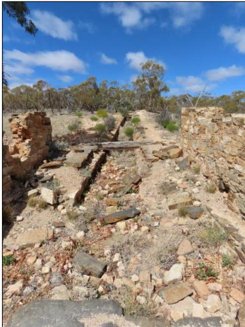
73. 50 m flue with collapsed roof looking towards collapsed chimney.
