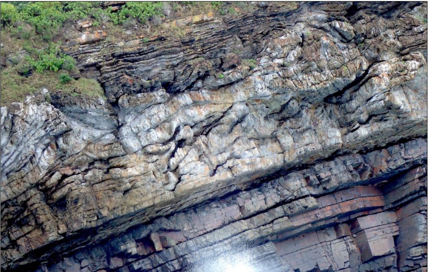
22. Skeletonized ignimbrite band weathered by the harsh marine environment removing softer material within the ignimbrite, accentuating the visual effects of the folds and deformities within the band. Note pelagic sediment layers above the ignimbrite.
