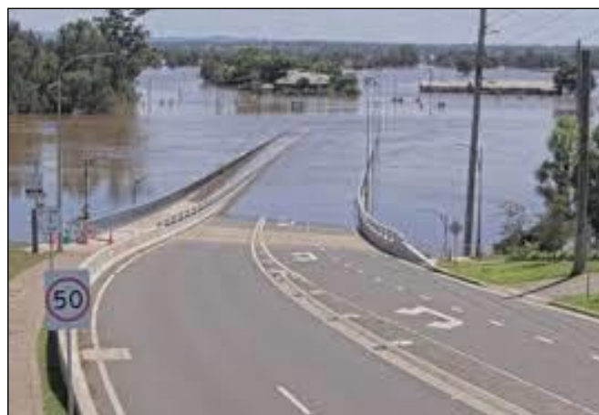
10. The replacement “flood free” bridge at Windsor. (Source: Blue Mountains Gazette).
