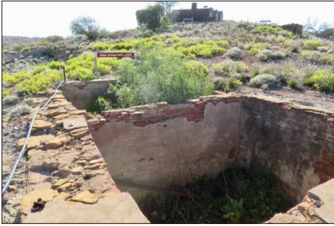
40. The water storage tanks at Blinman Copper mine.
