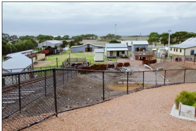
7. Buildings at Wonthaggi Coal mine.
