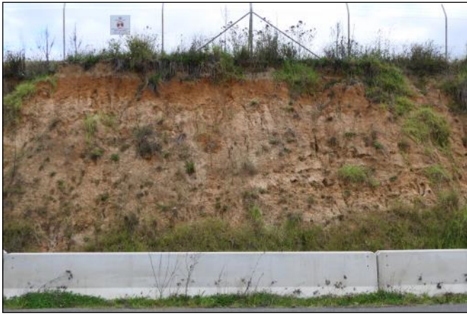
6. Profile of Londonderry Clay near Richmond RAAF Base. (photo Ron Evans).
