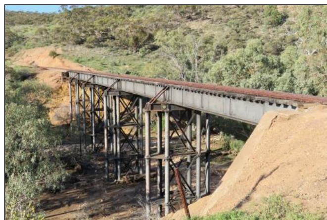
3. Plate Girder bridge near Woolshed flat.
