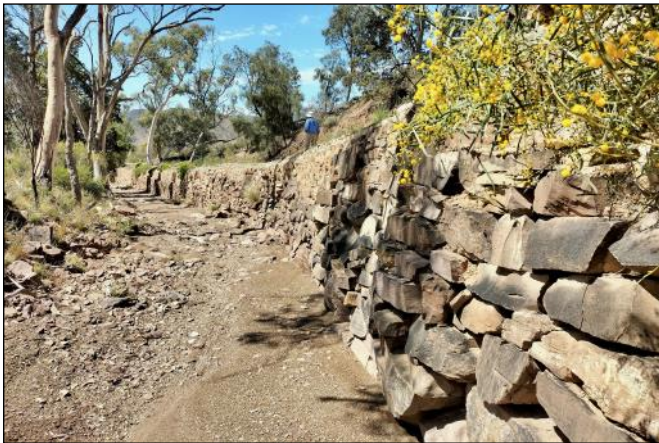
51. Dry stone wall long Glass Gorge Drive.
